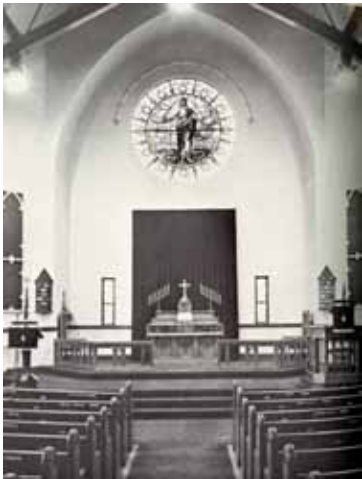
1956 – You can see the roof beams which will be revealed again, and the rounded profile of the pews and chancel.
