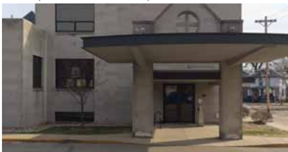
Westminster Presbyterian's main entrance on the west side of their building is where we will enter for worship.
